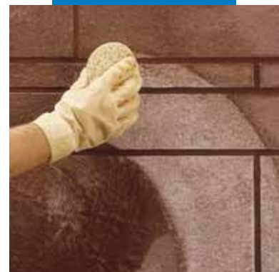
Cleaning and finishing the tile joints with a sponge
