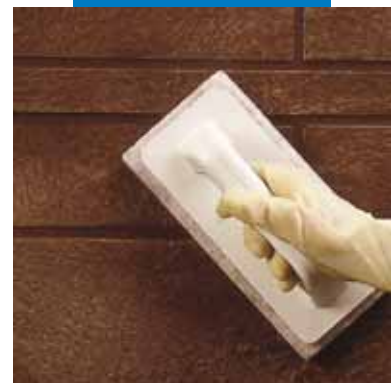
Cleaning the joints with Scotch-Brite® (when the product is partially set)
