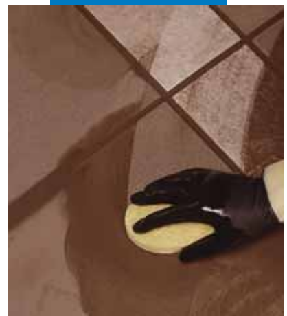
Cleaning and finishing the tile joints with a sponge
