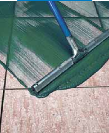
Spreading Ultracolor Plus on a floor with a rubber squeegee
