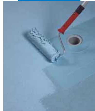
Application by roller of Mapelastic® AquaDefense second coat
