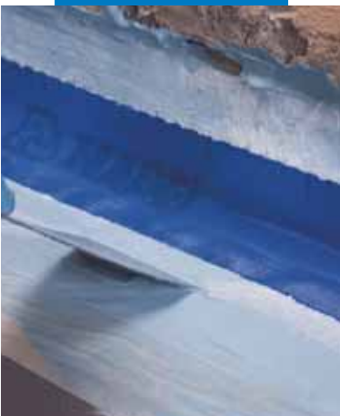
Application of Mapeband on a wall-floor fillet joint with Mapelastic® AquaDefense
