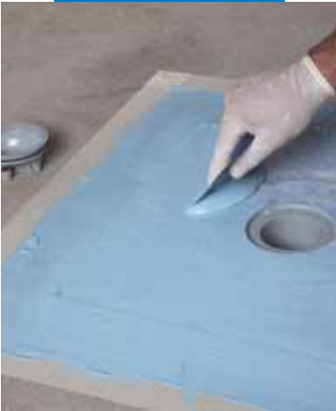
Impregnating Drain Vertical fabric with Mapelastic® AquaDefense
