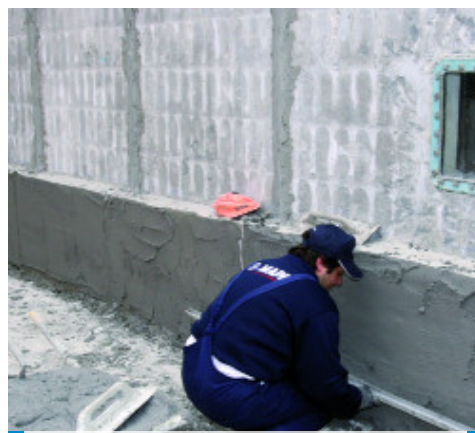
Levelling with a laying-on trowel
