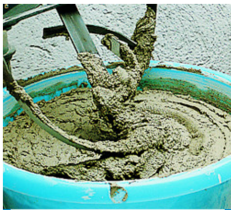
Mixing with a mini cement-mixer
