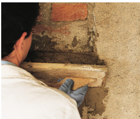
Application of Nivoplan with a float
