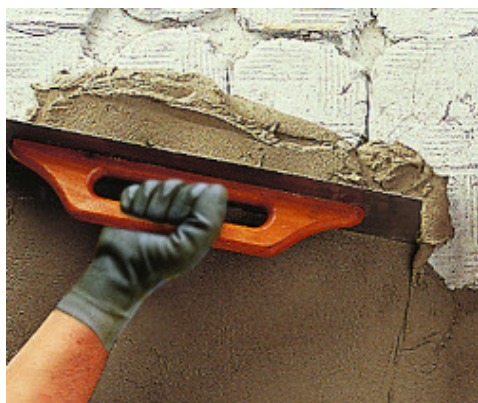
Levelling off the render with a straight-edge
