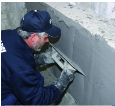
Restoring old brickwork
